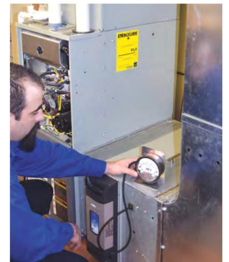
This time, the technician demonstrates taking the return duct pressure.
