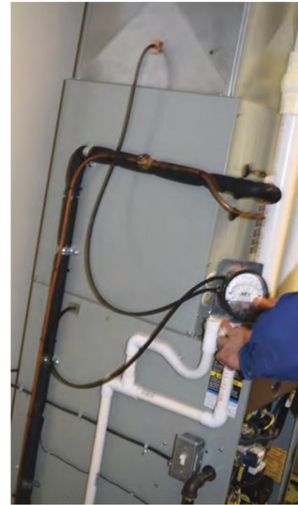
Technician demonstrates where to take coil pressure drop readings.
