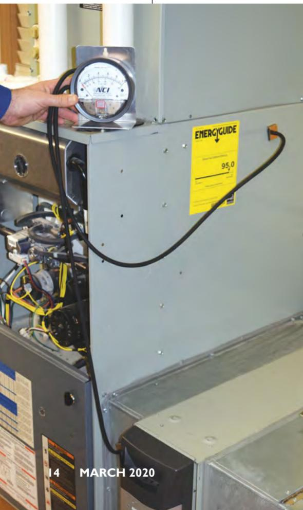
where air exits supply registers or enters return grilles, is near 0" w.c., a single point measurement identifies supply or return duct pressure.
