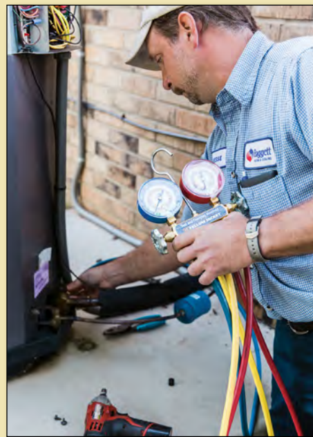
After static pressure and airflow testings, Jesse Waldrop tests refrigerant pressure to make sure the system performance is at its best.
