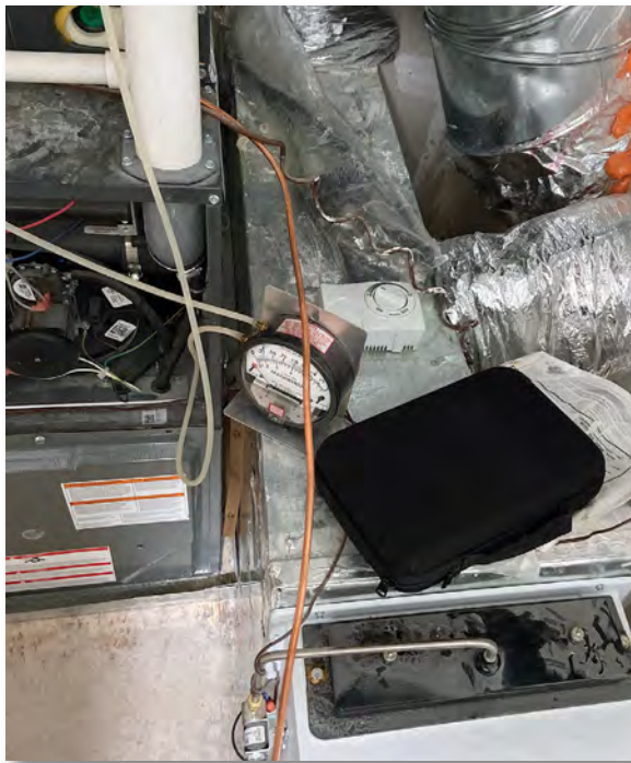
Diagnostics testing includes taking static pressure and temperature drop measurements, among several other tests.
