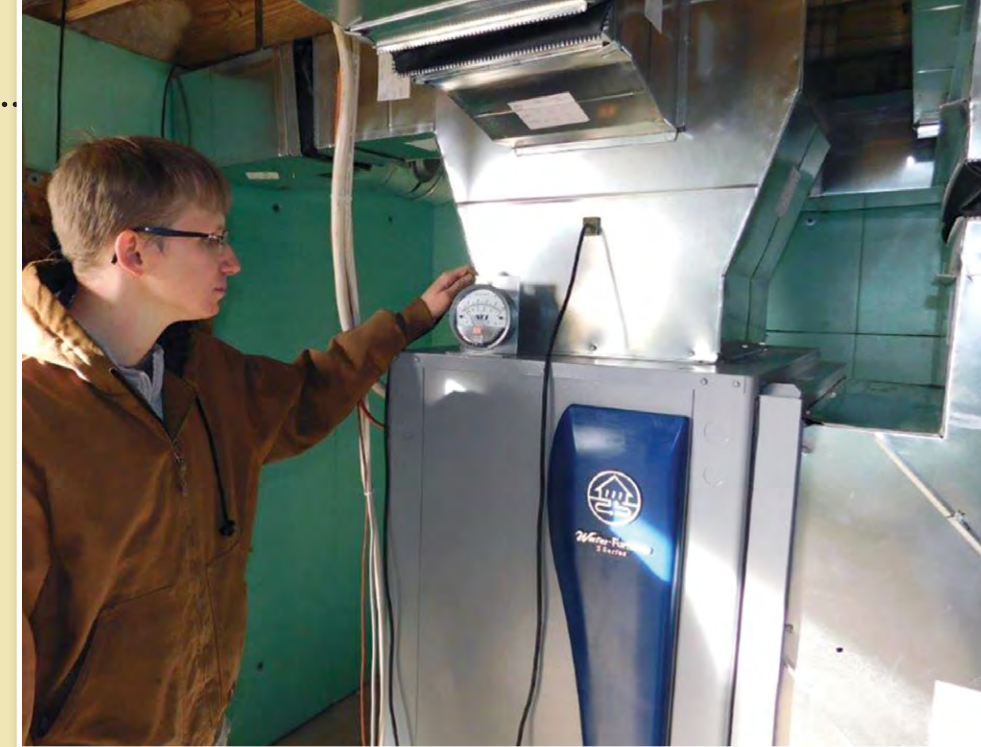
Senior Tech Dustin Kuzar performs a static pressure test on a geothermal unit.
