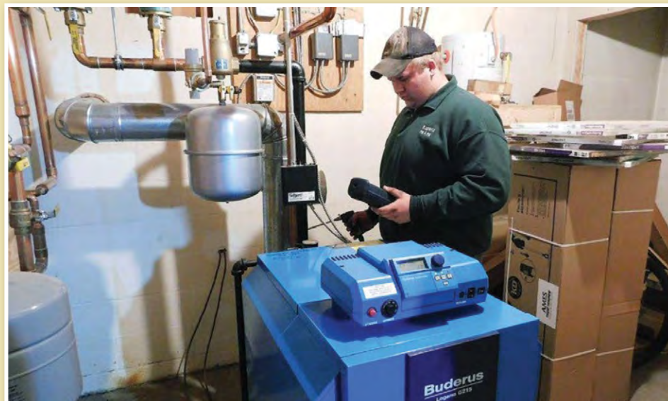
Kupetz technician Nate Martin conducts combustion testing on a residential boiler.
