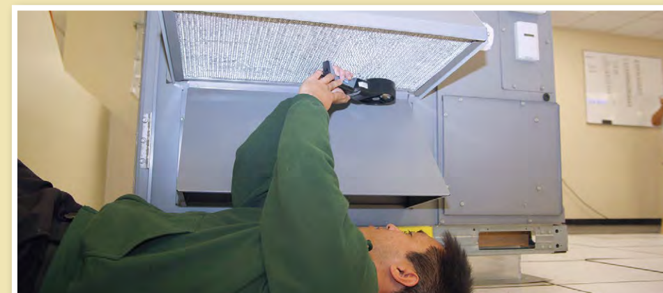
This student is performing a travers of an economizer intake using a rotating vane anemometer.
