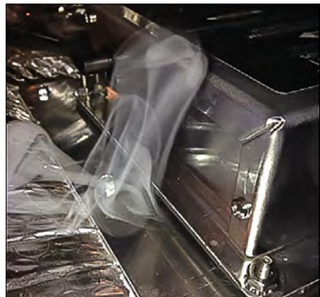
Using smoke showed that the newly installed filter rack created more problems than it solved.
