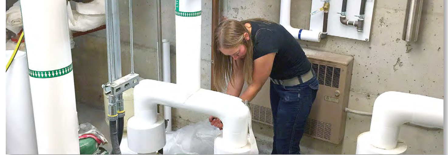
Working on balancing a commercial hydronics system.
