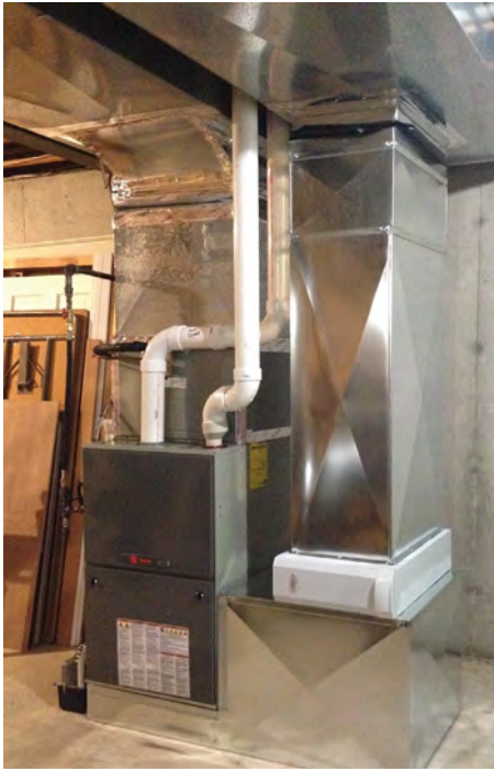
Figure 2: Second Example of Enlarging the Return Drop.
