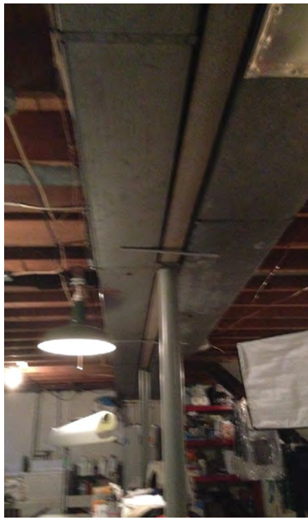
Figure 3: Increase Return Duct Size - Before.
