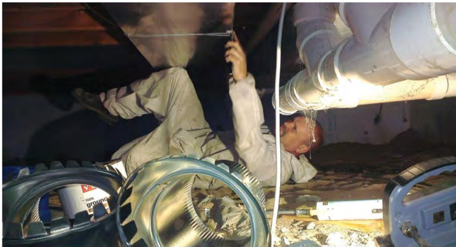
Duct renovations are an important part of the Schaafsma Performance-Based Contracting™ approach to HVAC service. [For more on this company, click here](#)
