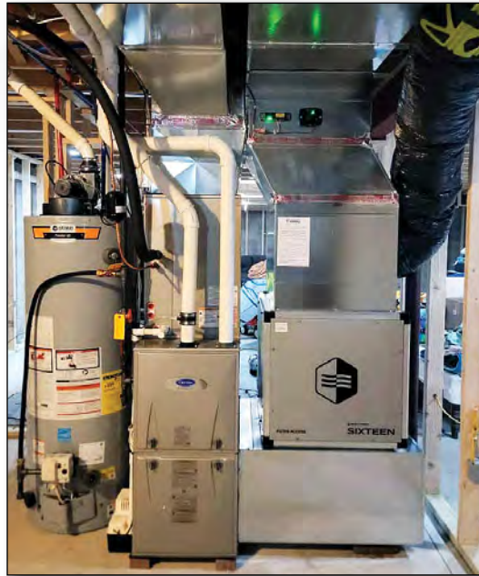
A system with a filter upgrade, showing a Dust Free Sixteen filter (MERV 16) installed.
