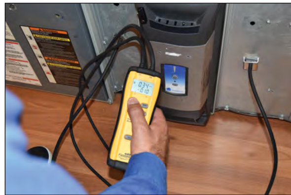
The cornerstone of High-Performance HVAC™ is conducting static pressure testing.
