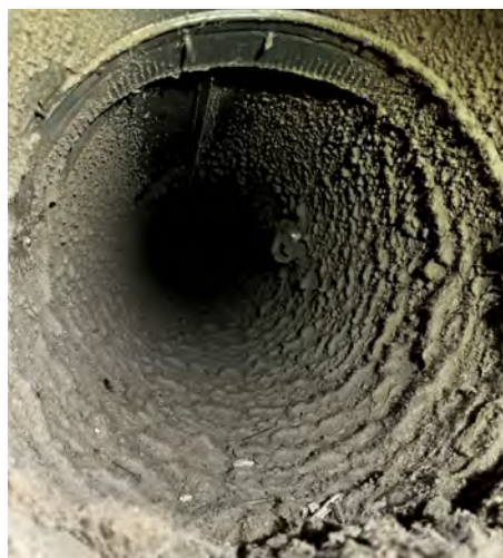
Example of the microbial and other growth inside ducts.
