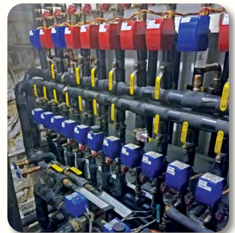
Dozens of low and high-temperature zone valves are meticulously mounted to a rack on the wall.
