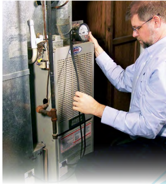
David Richardson demonstrates doing a static pressure test
