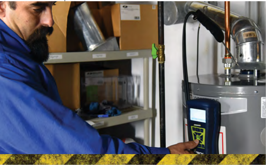
HVAC technician conducts a carbon monoxide draft test on a domestic hot water heater.
