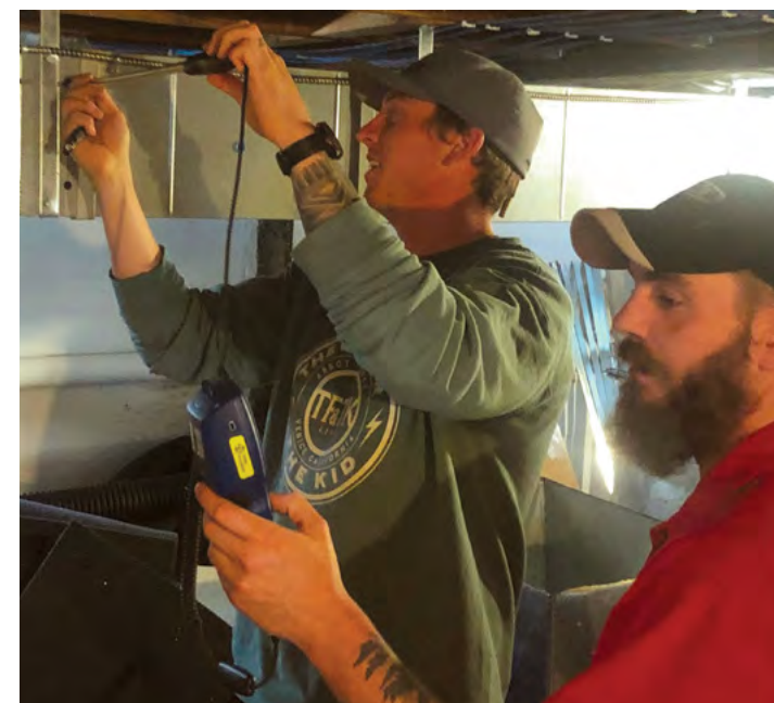
HVAC technicians testing airflow, velocity, and temperature in a commercial duct run.
