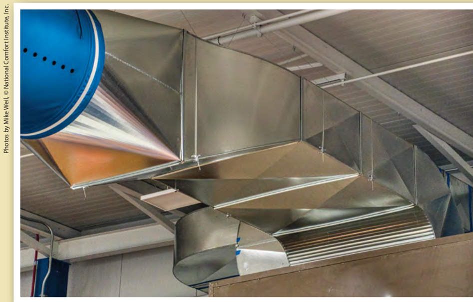
This is an example of the high-quality fabrication that Viccarone brings to the table. This is a commercial duct radius.
