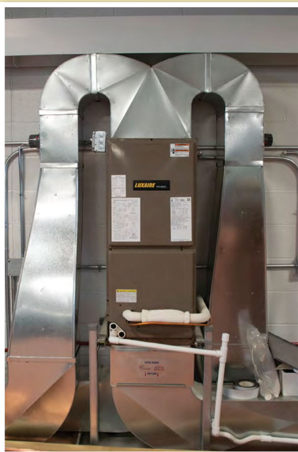
Pictured is a standard Viccarone furnace installation using custom-made inside/outside radius plenums for optimal airflow.
