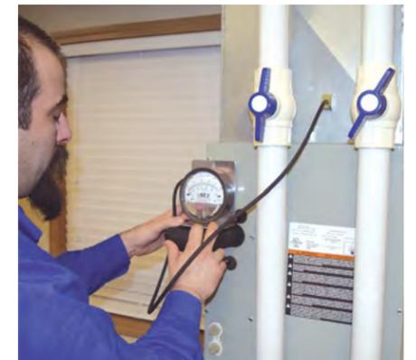
Technician demonstrating where to take supply duct pressure measurement.
