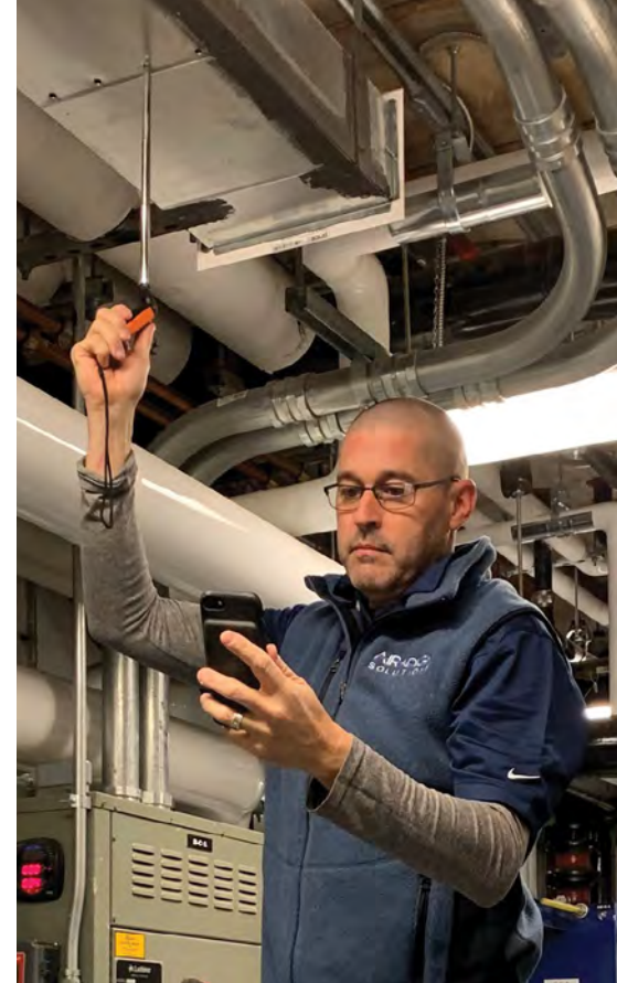
An Airadigm Solutions technician uses a hot wire to take a traverse in a mechanical room. This tool does not read negative numbers which could make your reading inaccurate.
