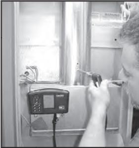
By checking combustion and draft he can unveil serious safety issues stemming from venting and combustion air deficiencies, even mechanical problems. He can also find serious efficiency problems resulting from improperly adjusted burners and other defects.
